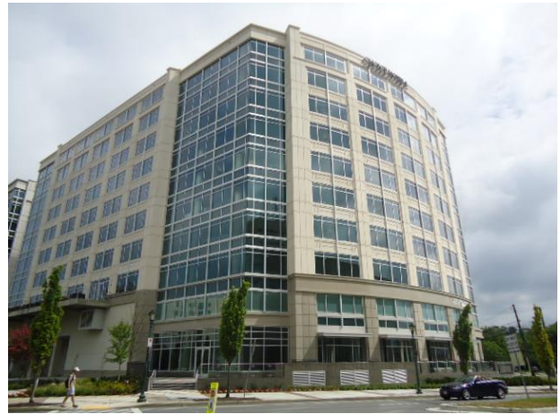
Figure 1: South West Corner – by JMV
